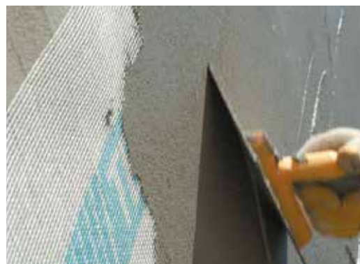
Embedding Glass Fibre Mesh
